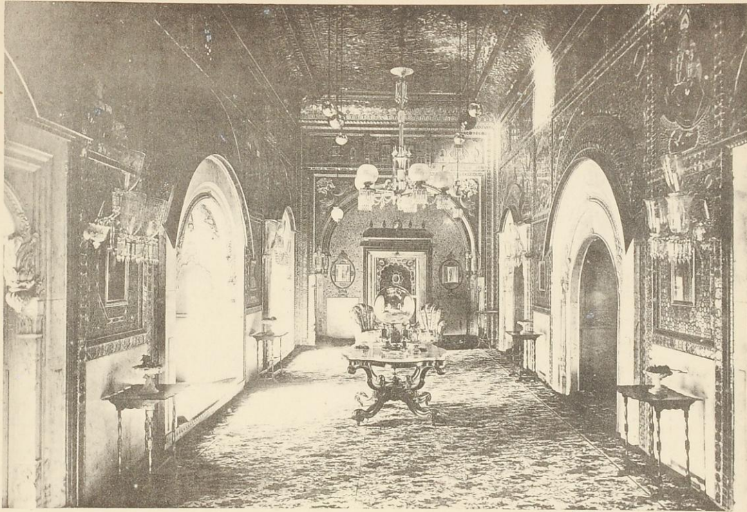
HALL AT BACK OF CITY PALACE, ULWAR.
